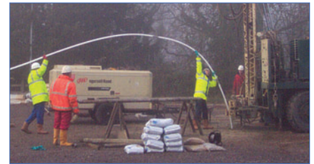
CMT Installation at UK Chlorinated Solvents Site (Source: Waterra, UK)
